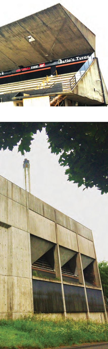
er house, Melrose; top: stadium for hels; left: former Bernat Klein studio
